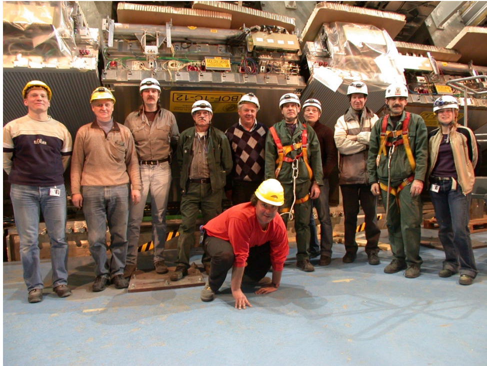
February 2005: Feet sector installation
