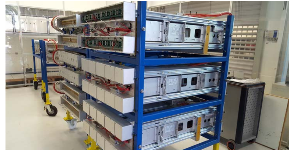
Completed BMG chambers for early 2017 installation
