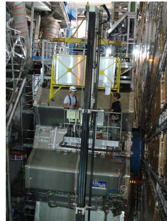
Installation of two 8-layer chambers in the bottom barrel sector in 2014
